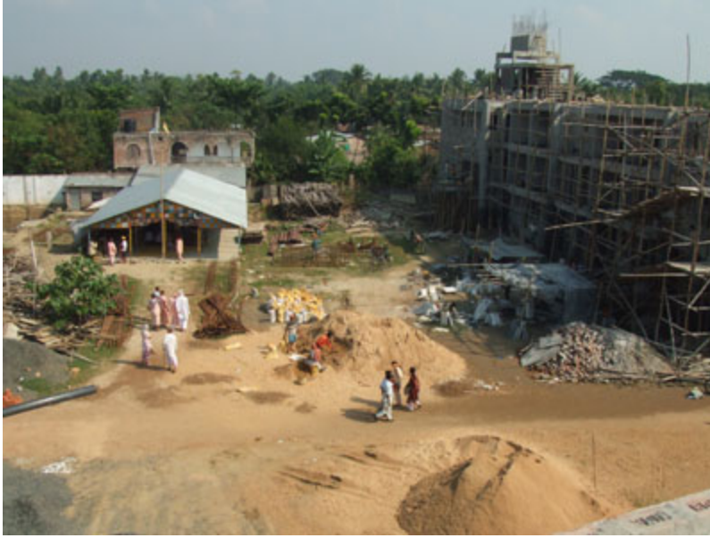
An overview of the temple construction.
